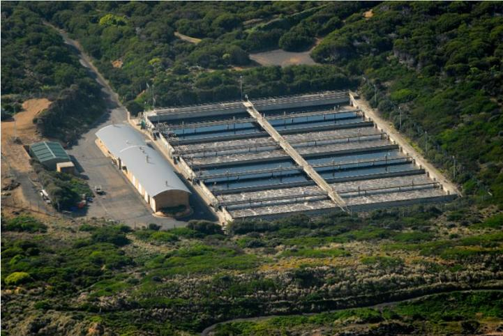
Like most treatment facilities across Australia, it has multiple systems in place to filter out the huge majority of foreign material that should not be disposed of down the toilet or drain. Plastics, baby wipes and other materials are screened out prior to entering the plant, but the equipment is not designed to remove tiny plastics such as nurdles.
