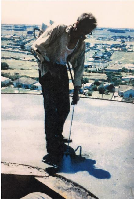
John Snaauw pouring concrete on top of the east tower deck during construction.
