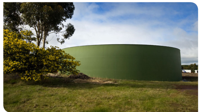
The clear water storage tank at the Hamilton Water Treatment Plant
