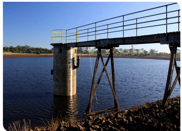
One of the storage reservoirs along the Hamilton pipeline route
