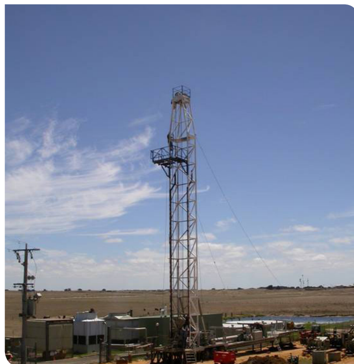
A bore used to source water from deep within the Dilwyn Aquifer
