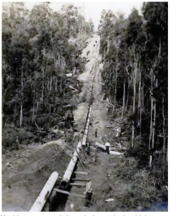
Machinery was crude by today's standards with horse drawn scoops, ploughs and drays used together with tractors. Trenches were dug by hand where the terrain was too steep to use horses and scoops. A total of 300 men and 170 horses were used at the peak of the operation.
