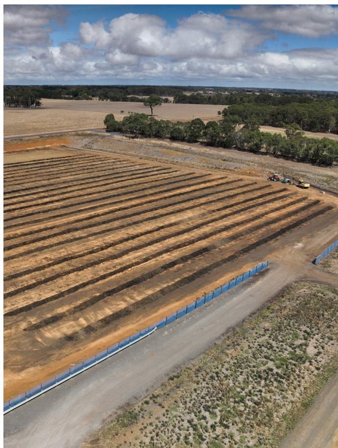
Biosolids drying area, Hamilton
